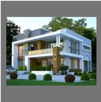
Civil Construction Contractors
