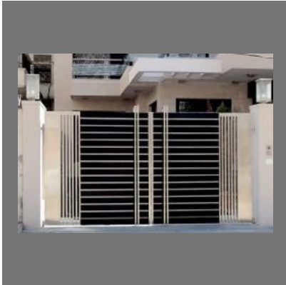
Stainless Steel Main Gate
