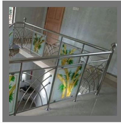
SS Staircase Railing
