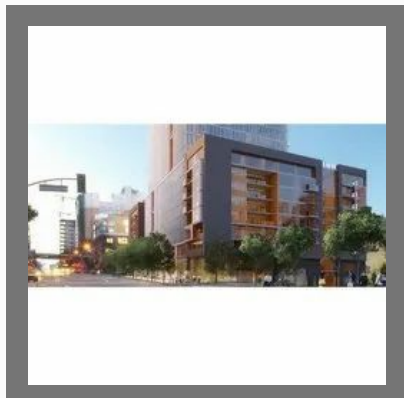
Residential Electrical Work
