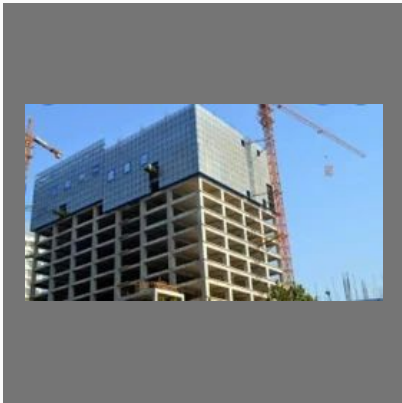
Commercial Mall Constructions
