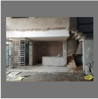
Guest House Construction
