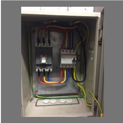
LT Cable Laying Services
