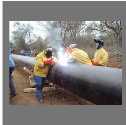
Gas Pipeline Work
