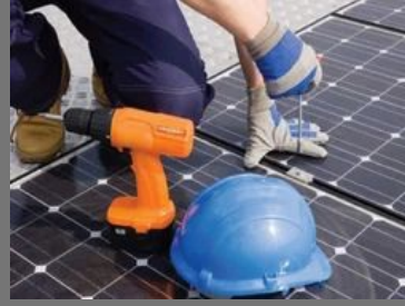
O & M PREVENTIVE MAINTENANCE SERVICES
