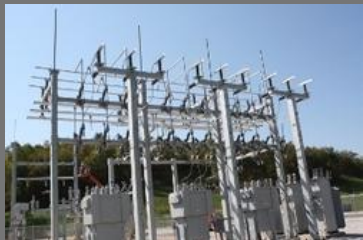
Substation Maintenance Services
