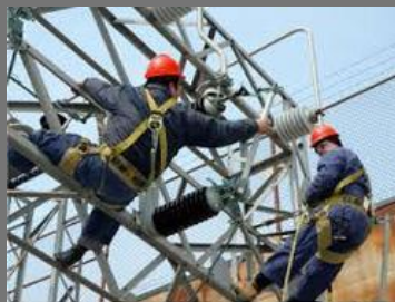
Substation Repairing Services
