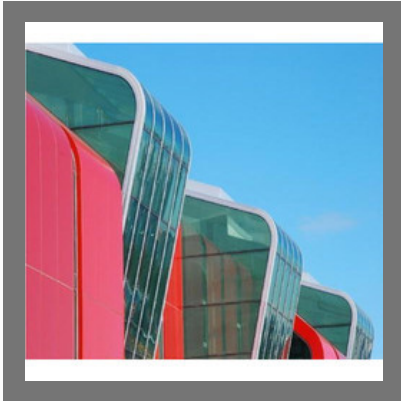
Bend Roof Glass
