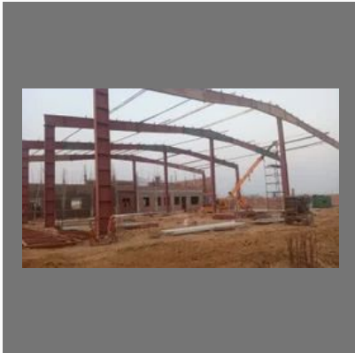
Industrial Shed Fabrication
