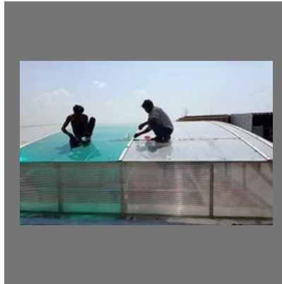
Polycarbonate Sheet Roofing Installation Service
