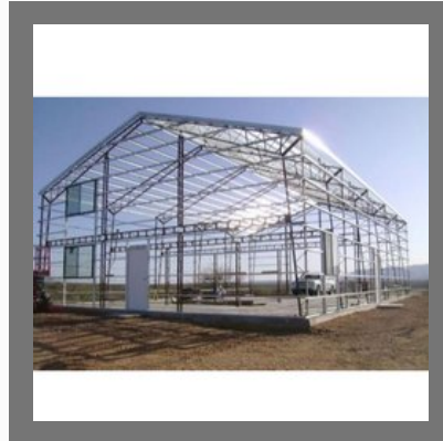
MS Industrial Shed
