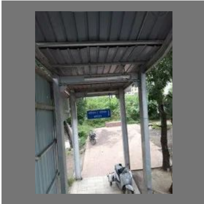
Foot Overbridge Construction
