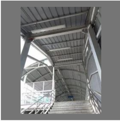
Footover Bridge Construction Services
