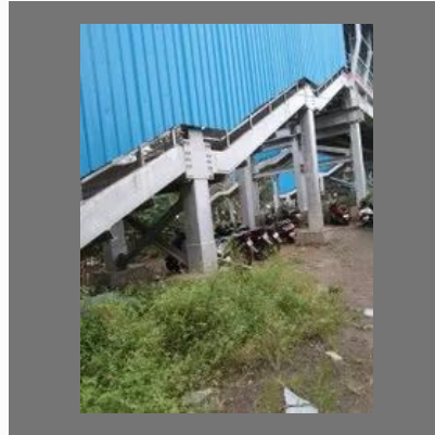
Foot Overbridge Construction
