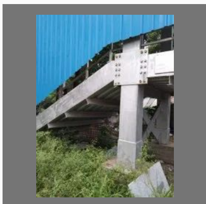
Foot Overbridge Construction
