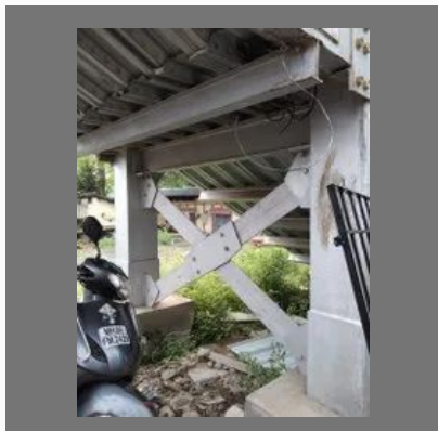
Foot Overbridge Construction
