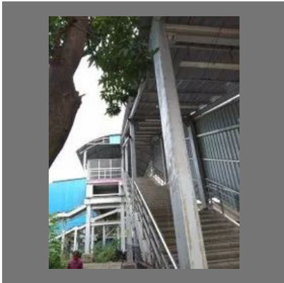
Footover Bridge Construction Services
