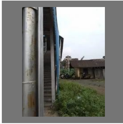
Footover Bridge Construction Services
