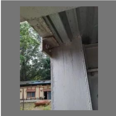
Foot Overbridge Construction
