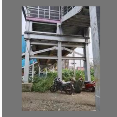
Foot Overbridge Construction
