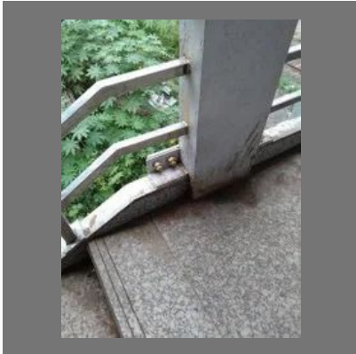
Foot Over Bridge Construction Services
