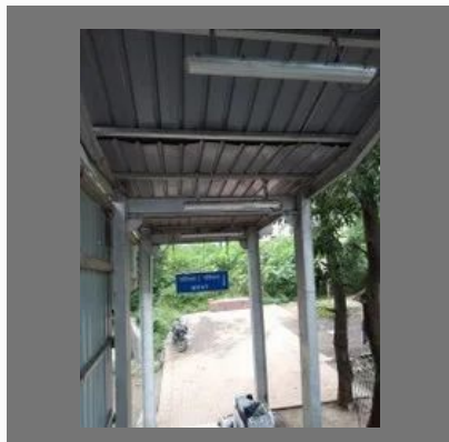
Foot Over Bridge Construction Services
