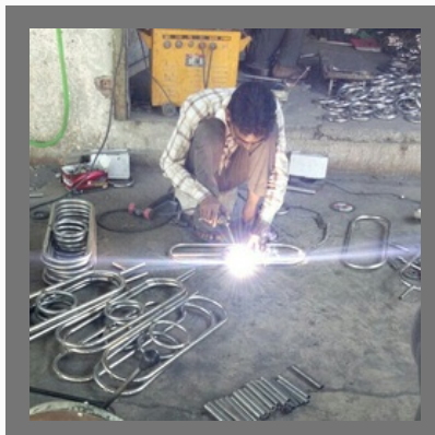
Steel Railing Fabrication Work
