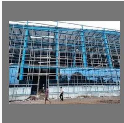
Factory Shed Structure Fabrication Service
