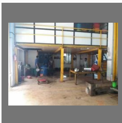
RCC Gala For Rent In Chinch Pada Naka Vasai East
