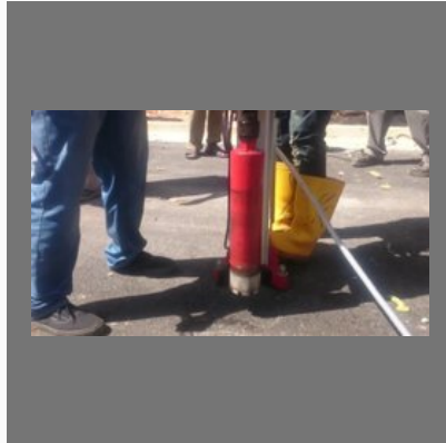
Bitumen Core Cutting
