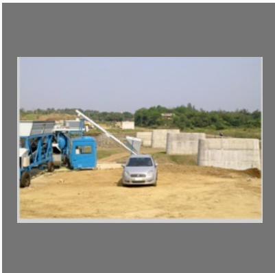
Varoli River Bridge Construction
