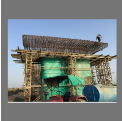
Nargol Creek Bridge Construction
