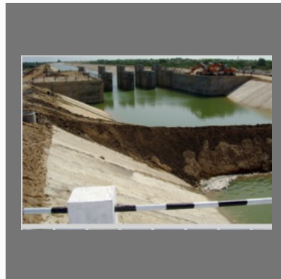
Ujjainwada Narmada Canal Bridge Construction Service
