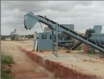
Road Construction Service
