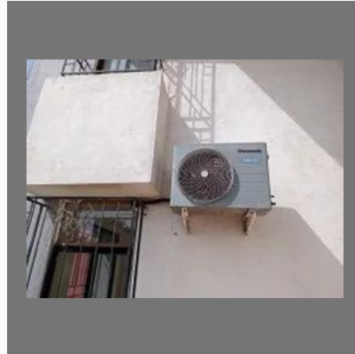
Split Systems Installation
