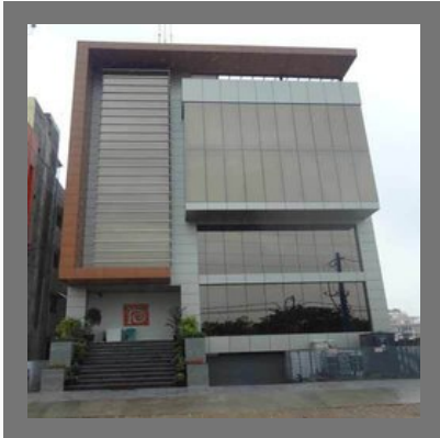
ACP Fabrication Service
