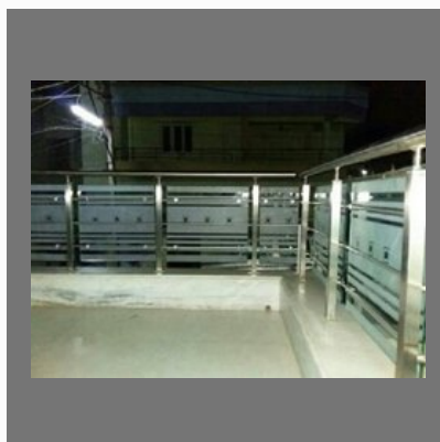
SS Glass Roofing Railing
