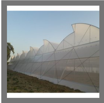
Naturally Ventilated Polyhouse
