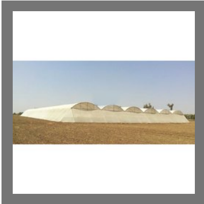
Shade Net House Structure
