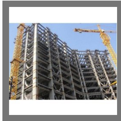
Commercial Buildings Construction Service
