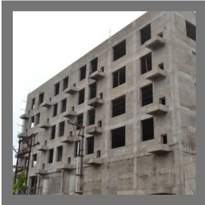
Apartment Construction Services
