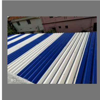
Colour Roofing Shed
