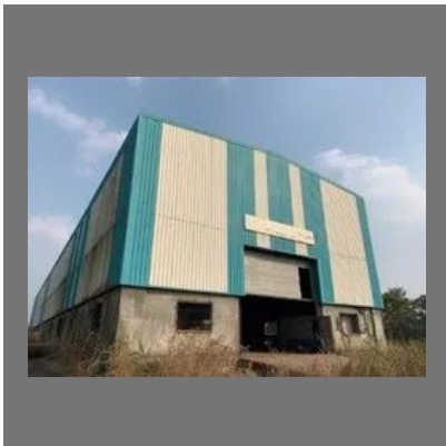
Industrial Prefabricated Factory Shed
