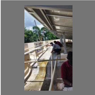
All Plumbing Work
