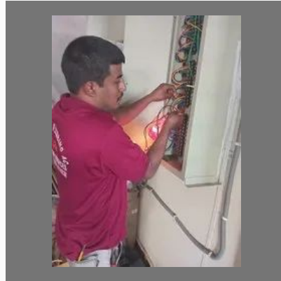
Electrical Items Repairing Services
