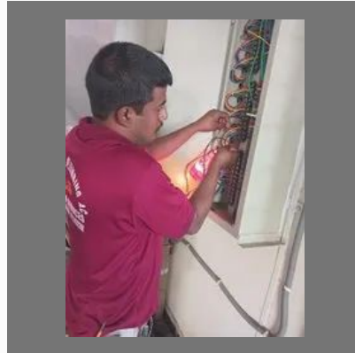
House Wiring Work Services
