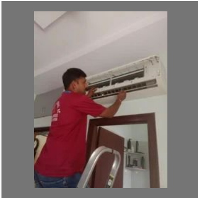
Split Ac Installation Services
