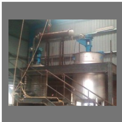
Alkyd Resin Plant
