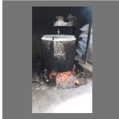
MS Mixing Tank
