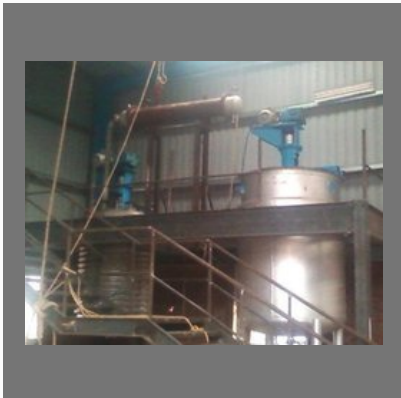
Alkyd Resin Plant
