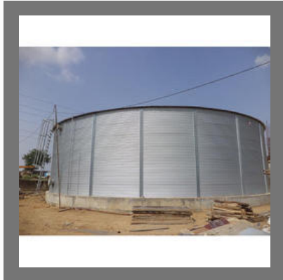
Bolted Panel Water Tanks
