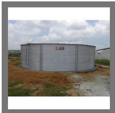
Rain Water Harvesting Tank
