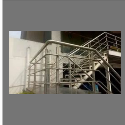
Stainless Steel Railing
