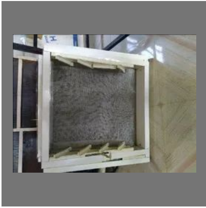
Washroom Window Frame
