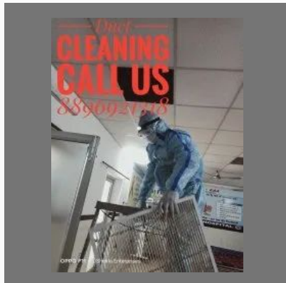
Robotic Duct sanitization Service
