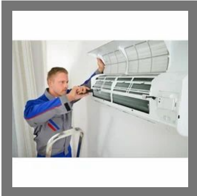
Air Conditioner Maintenance Service
