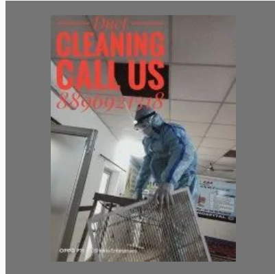
Duct Sanitization Service
