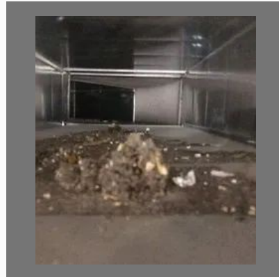
Duct Cleaning Services
