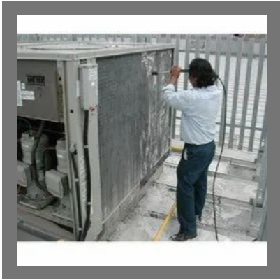
AHU Duct Coil Cleaning Services
