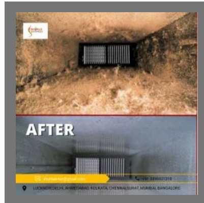
Laundry Exhaust Duct Cleaning
