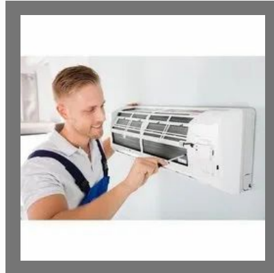
Air Conditioning Repairing Service
