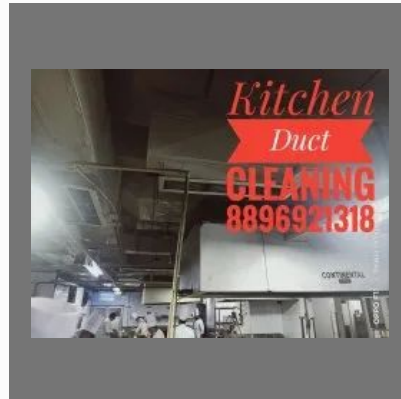
Kitchen Duct Cleaning
