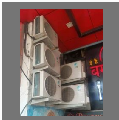
All Types Ac Installation And Service
