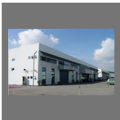
Building Construction Project
