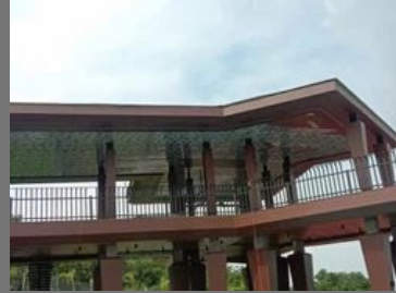
Acp Cladding Work
