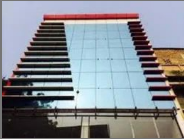
Acp Glass Glazing Work
