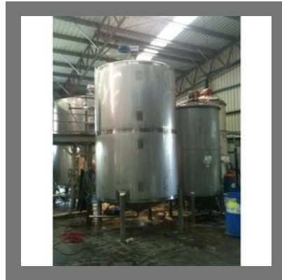
Oilment Cyrup Plant
