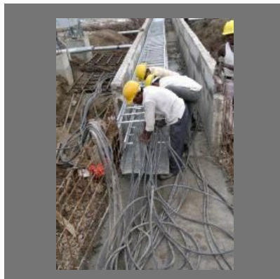
LT Cable Laying Service
