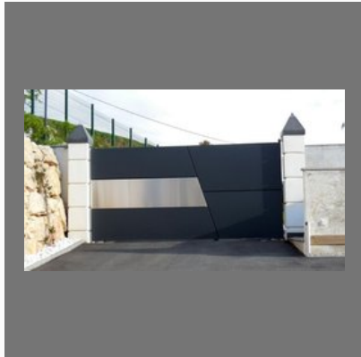
Motorized Sliding Gate
