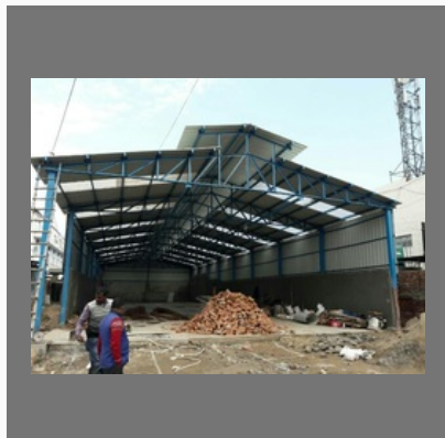
Industrial Iron Shed Structure
