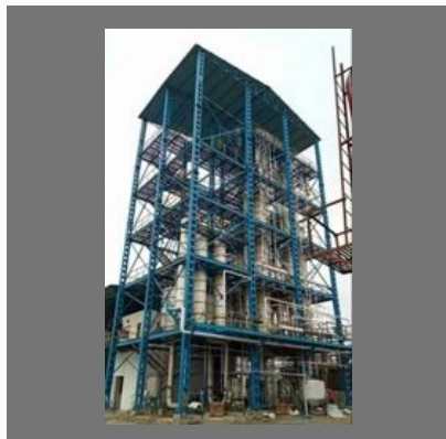
Fuel Ethanol Plant
