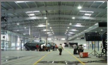
Industrial Building Construction Service
