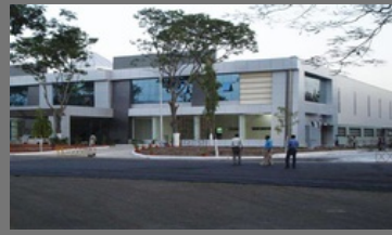
Commercial Building Construction Service
