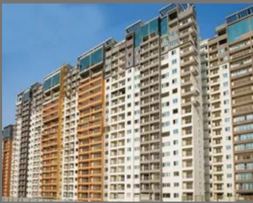
3 BHK Apartment Construction Service
