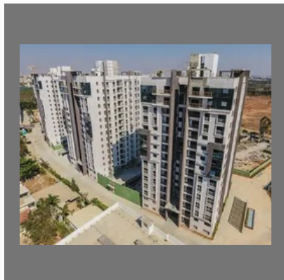
Residential Apartment Construction Service
