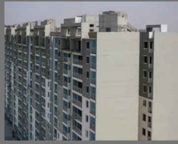
2 BHK Apartment Construction Service
