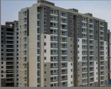
1 BHK Apartment Construction Service
