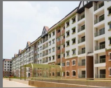
4 BHK Apartment Construction Service
