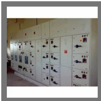
DG Set Panel Repair Service
