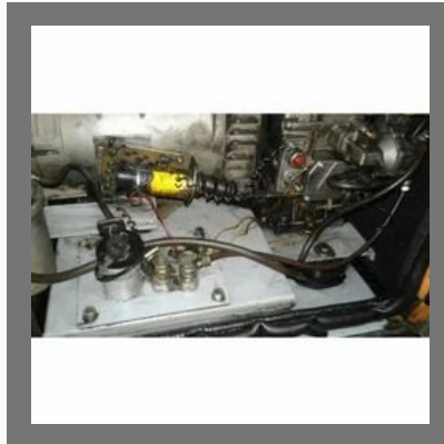
DG Set Generator Maintenance Service
