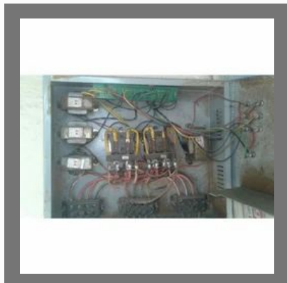
Genset Panel Repair Service
