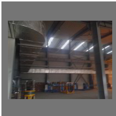
Industrial Ducting Work
