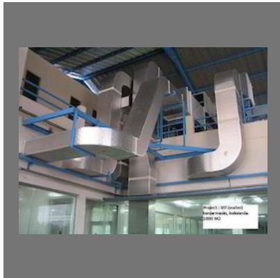
Pre Fabricated Duct
