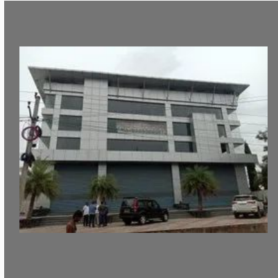
ACP Sheet Wall Cladding Service
