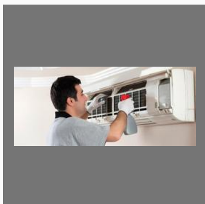
AC Installation Services
