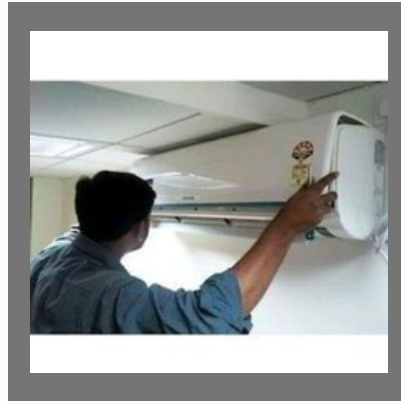
Air Conditioner Maintenance Services
