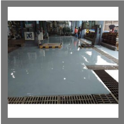
Epoxy Flooring Service
