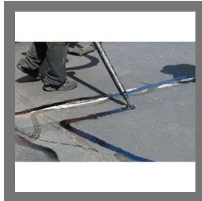
Crack Filling Service
