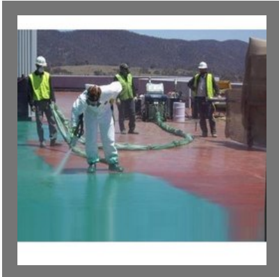
Industrial Waterproofing Services
