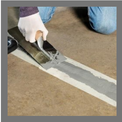
Expansion Joint Treatment Service
