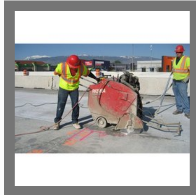
RCC Road Groove Cutting Service
