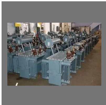
Transformer Repairing Service
