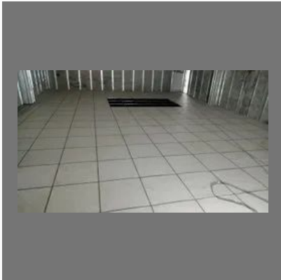
Steel Cementitious Bare Raised Access Floors
