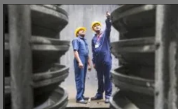
Energy Management Service
