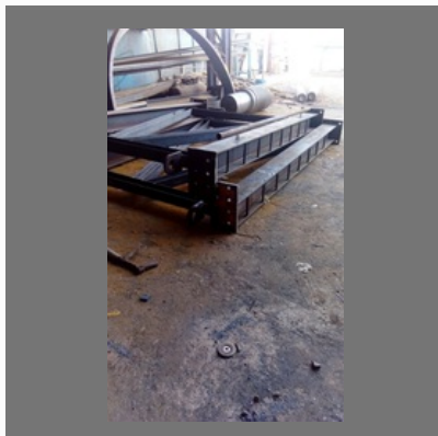
Heavy Shed Fabrication
